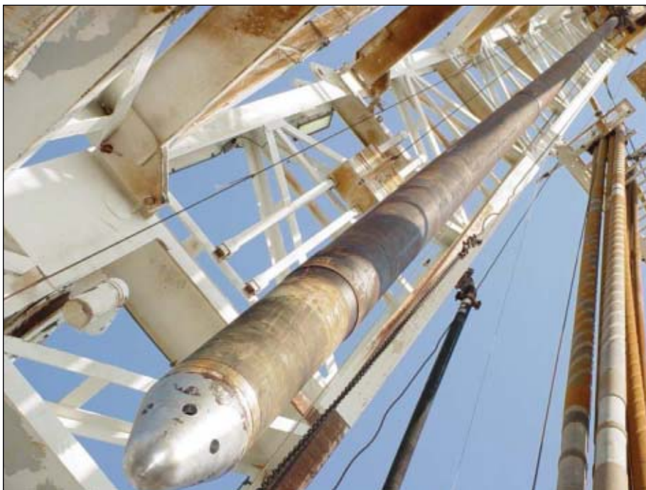
Prior to expansion, the linEXX assembly hangs in the derrick, as illustrated in this field trial application (Fig. 1).
